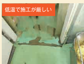
冷凍庫・冷蔵庫の床
